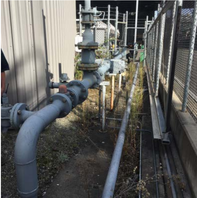
Natural Gas Line Provided with SGSV
